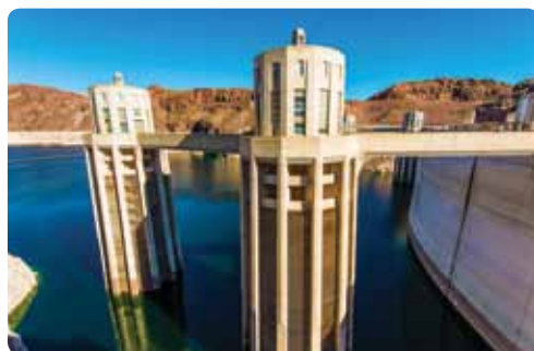
Hoover Dam intake towers
